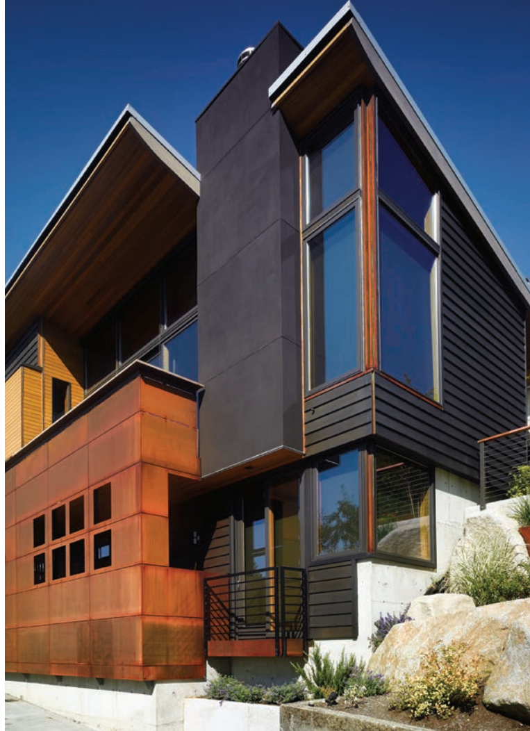
PHOTO BY KEN GUTMAKER / COURTESY OF RES ARCHITECTURE+DESIGN
