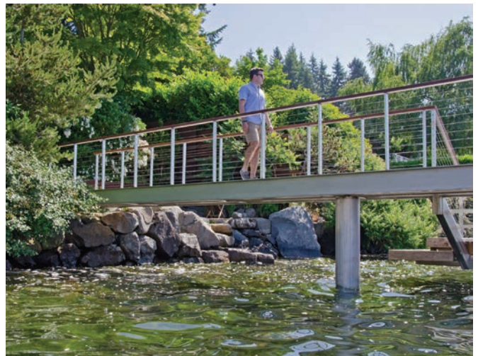
Meydenbauer Bay Bridge / Builder: Tend Home Services
