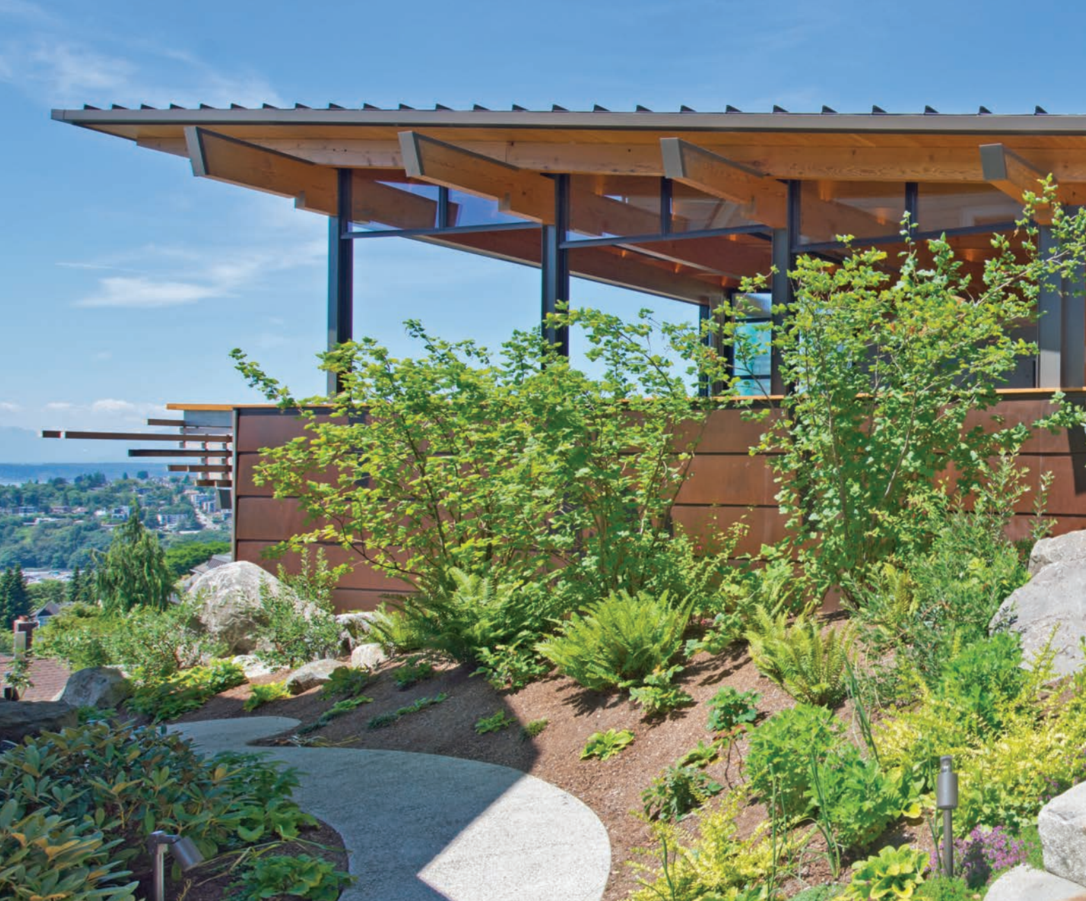
Queen Anne Pavilion, Seattle | Builder: Krekow Jennings | Metal Fabrication: Architectural Elements
