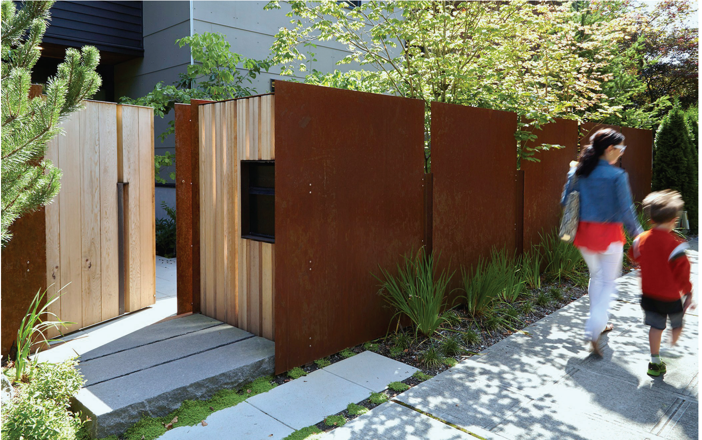
Steel fence panels. Rusted with apple cider vinegar. Finished with boiled Linseed Oil. Madison Park Garden by Robert Edson Swain, Architecture + Design. Contractor: Krekow Jennings Patina Fabrication: Architectural Elements. Photo: Ken Gutmaker
